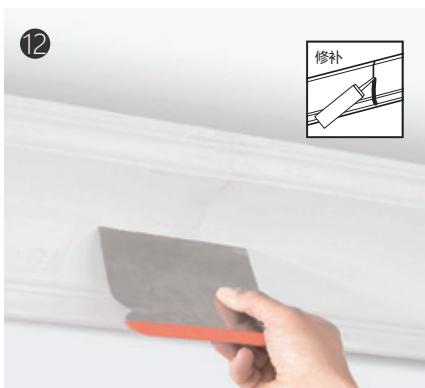
使用水性原子灰修补缝隙 Repair gaps with water-based putty
