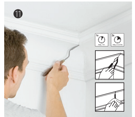
擦除连接处溢出的胶 隔2-3小时擦除一次，使用丙酮清洗 Wipe the glue overflowing at the connection, wipe it every 2-3 hours, Clean with acetone
