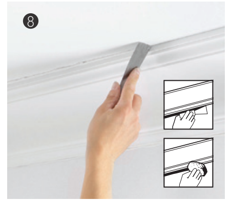
用海绵擦除溢出的胶水 Use a sponge to wipe off the spilled glue
