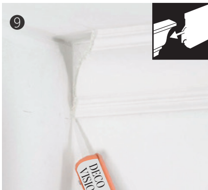
在连接处涂上西卡胶 Apply Sika Glue to the joints
