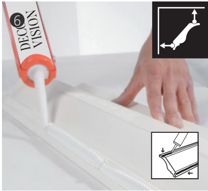
在贴胶面涂满西卡胶 Apply Sika Glue on the adhesive surface
