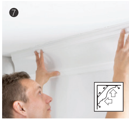
贴紧墙面安装 Close to wall installation
