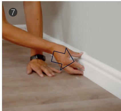
7 将线条贴紧安装 Install the lines tightly
