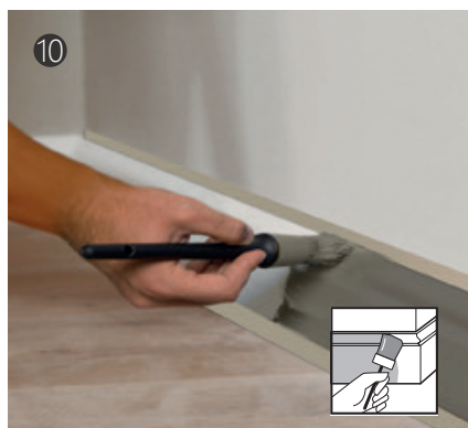
完成后就可以上色了 After finishing, you can paint
