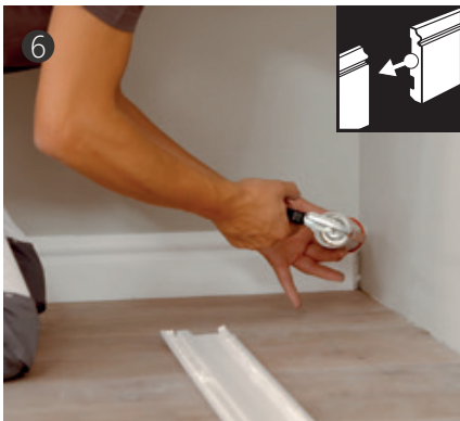
6 在连接处涂上西卡胶 Apply Sika Glue to the joints
